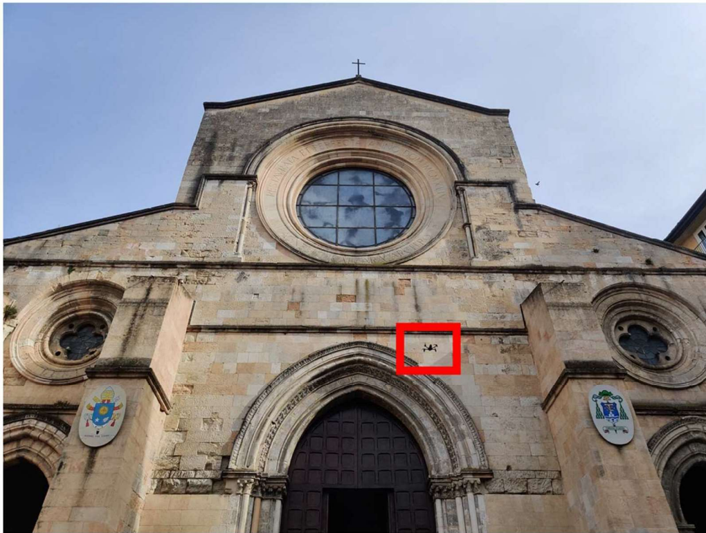
Figure 4. Detail of photogrammetric survey.
