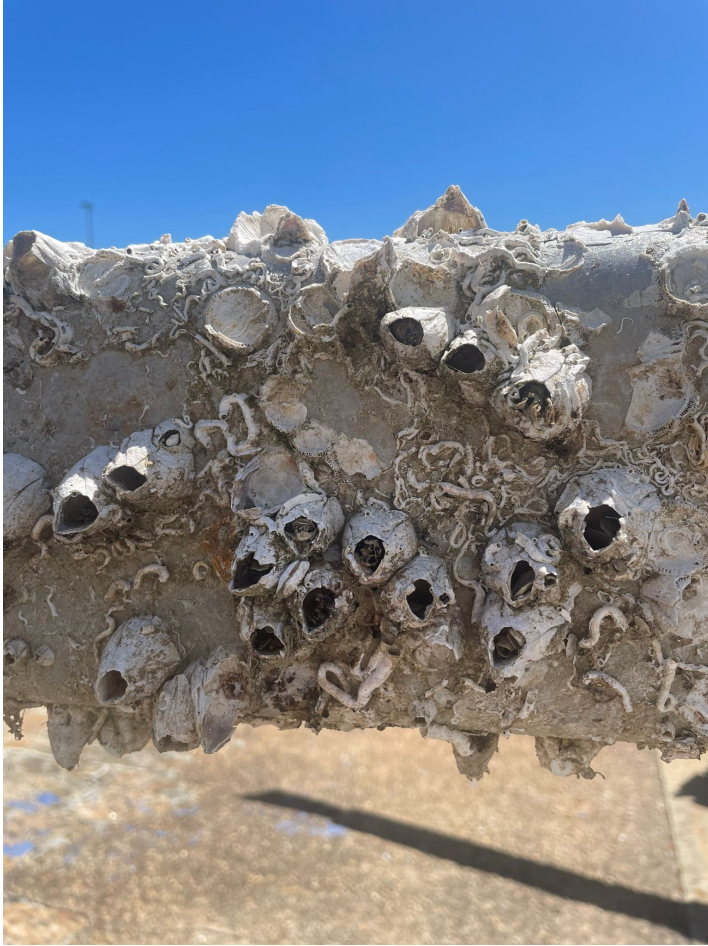
Figure 3.8: Real barnacles (“Balanus amphiprite”) on an iron structure in France.
