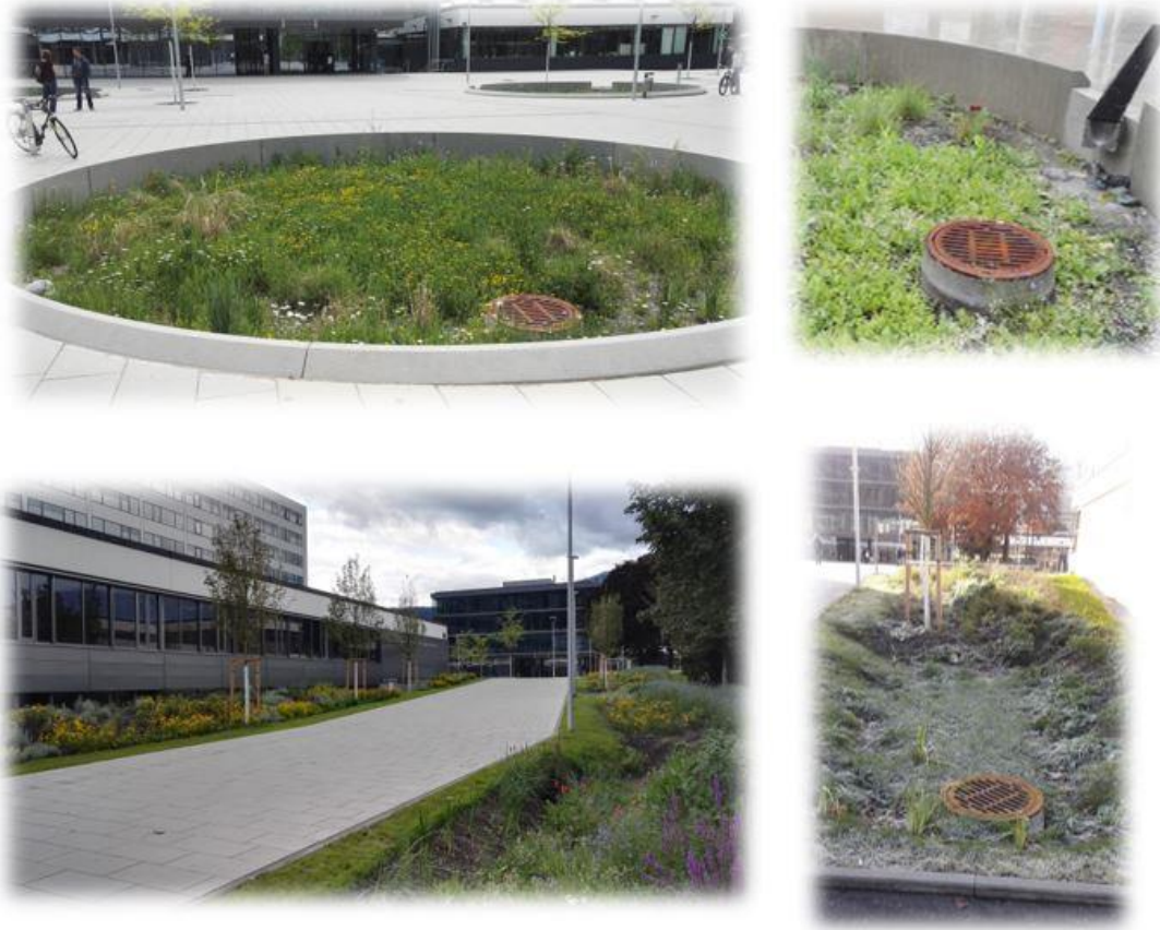
Figure 3.1: Pictures of the two different types of RGs at University Campus Innsbruck, the circular ones on the top, where is possible to observe the open channel too, and the semi-rectangular one, below.
