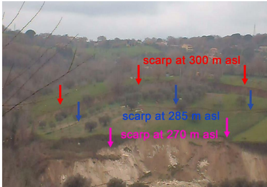
Figure 4.6 – The slip surface emerging at the elevation of 285 m a.s.l. (indicated by the blue arrows)
