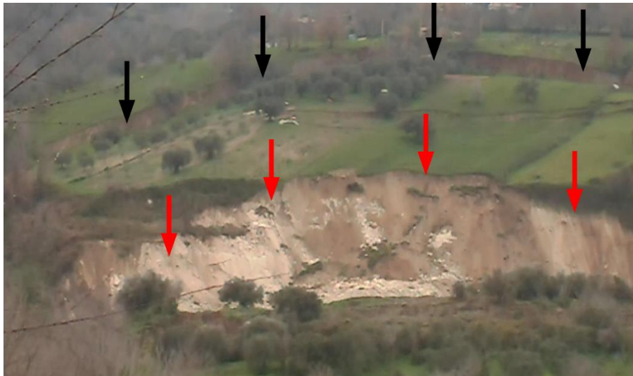
Figure 4.58 – Screenshot taken from a video filmed during the post-failure stage of the landslide, corresponding to the output plotted in Figure 4.57a (black arrows indicate the scarp at 300 m a.s.l., whereas red arrows indicate the scarp at 270 m a.s.l.)
