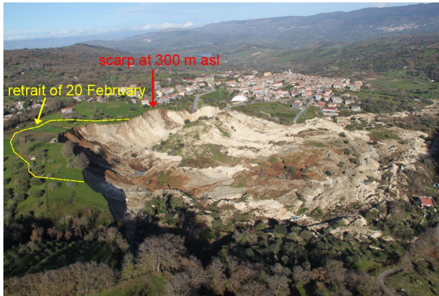
Figure 4.2 – Aerial view of the Maierato landslide
