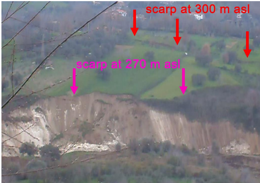
Figure 4.5 – The slip surface emerging at the elevation of 300 m a.s.l. (indicated by the red arrows)
