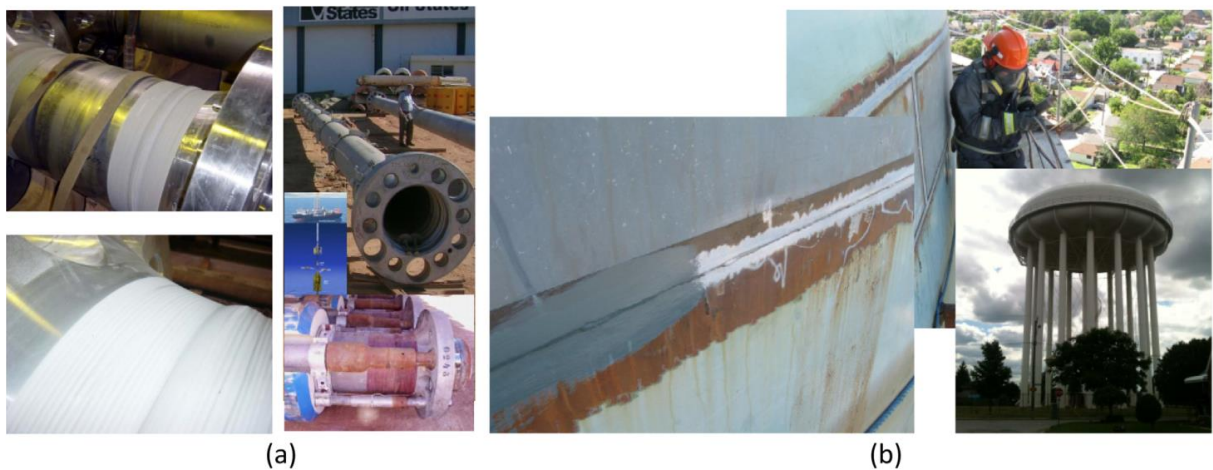
Fig. 1.20: Corrosion protection of deep water riser (a) or welded seams of large metal structures (b) produced by cold spraying [28]
