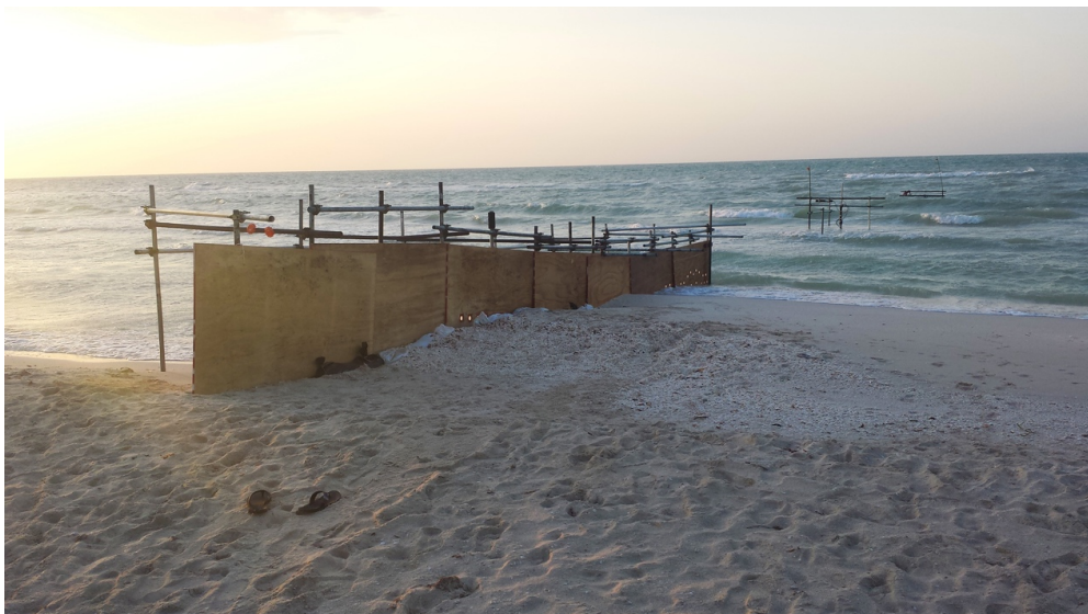
Figure 7.4 - Temporary groyne made of wood sections (Medellin et al., 2018)
